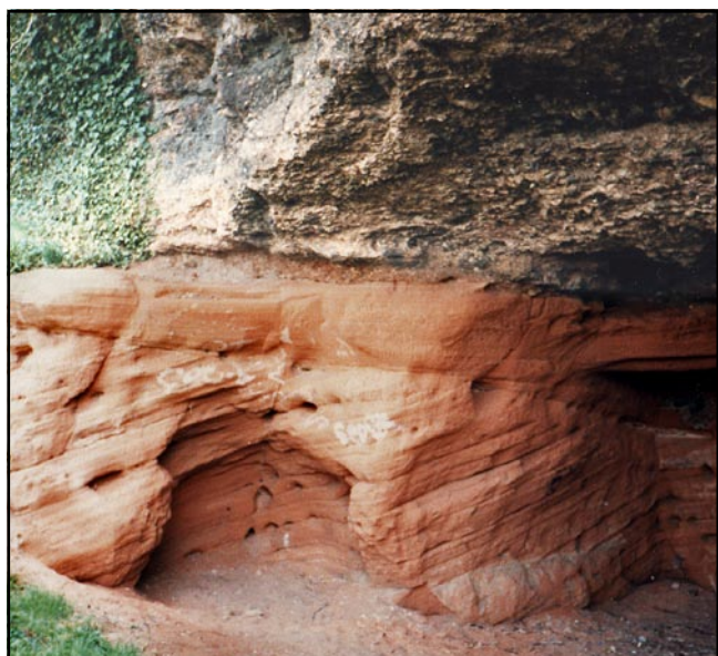
Two of the Hermitage Caves, in the dune-bedded Bridgnorth Sandstone with the Kidderminster Conglomerate above.
